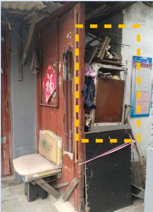
Messy clutter stored behind the door
